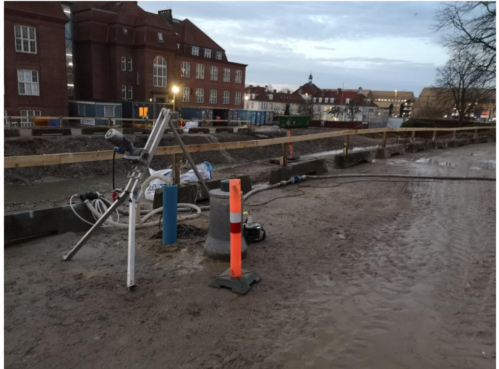
Figur 2-1: Billeder af pumpeboring.
